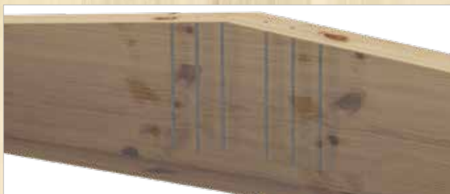
Reinforcement with screws in roof ridge area
