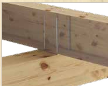
Reinforcement in the point of support
